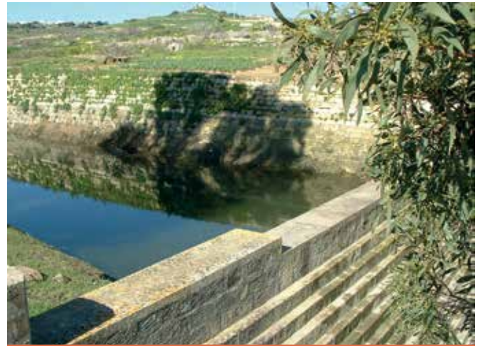
Freshwater is allowed more time to percolate into the aquifer by the building of dams in valleys, as well as by the digging of ponds, reservoirs and wells in the fields.
