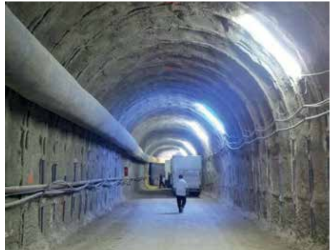
A 17-kilometre tunnel was dug under Attard, Balzan and Birkirkara in order to channel run-off rainwater. Rainwater which used to flood the streets is now finding its way into this tunnel and then to sea.
